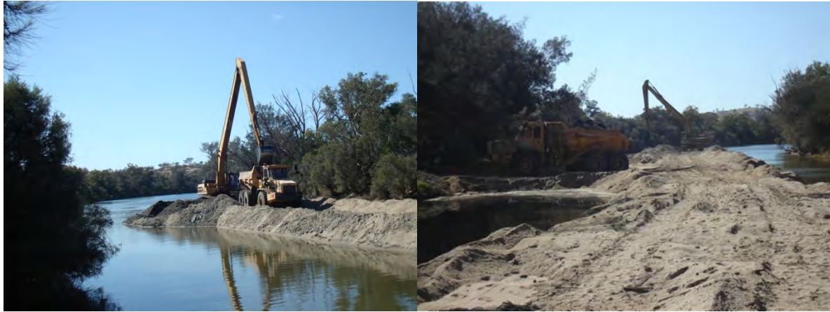
Figure 1. Removal of sediment from Gwambygine Pool in October 2010 (photos courtesy Wheatbelt NRM Inc).
