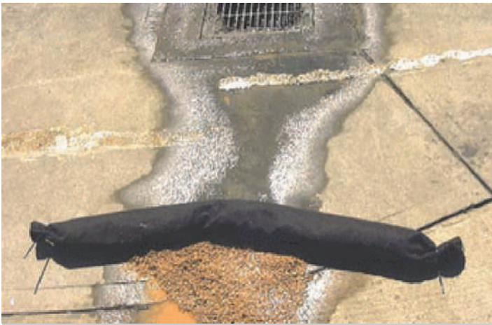
Y Fabric "sausage" may help to stop sediment entering stormwater drains
