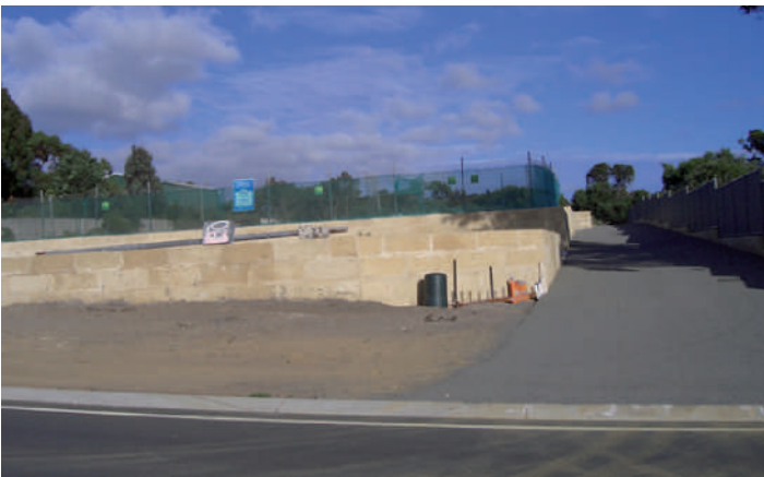
Y Stabilised entry / exit during construction
