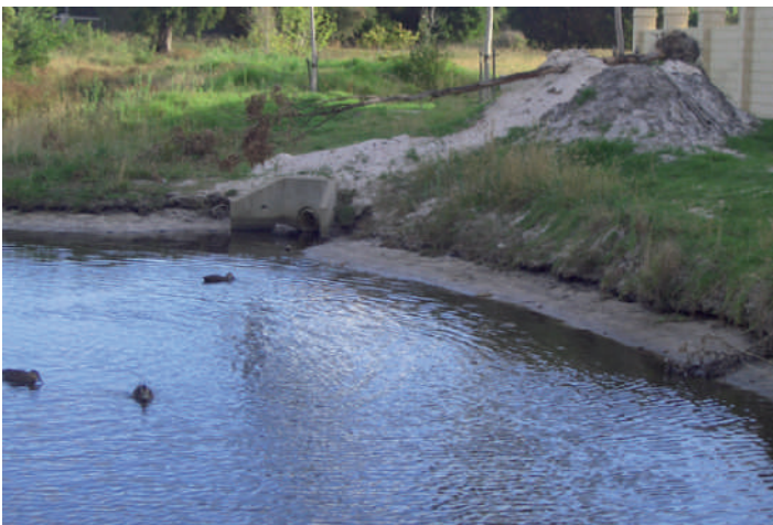
N Waste sand and rubble indiscriminately discarded onto side of creek
