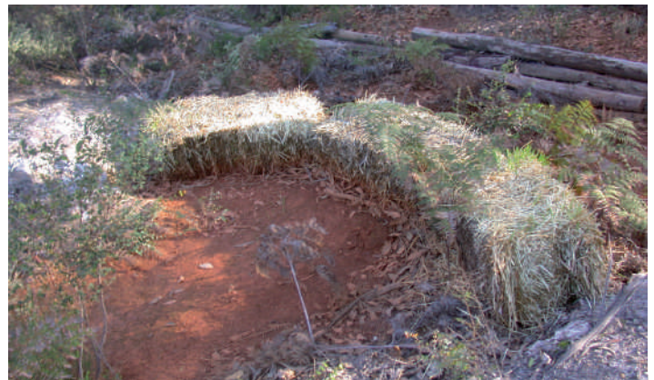
Y Hay bales used to restrict sediment
