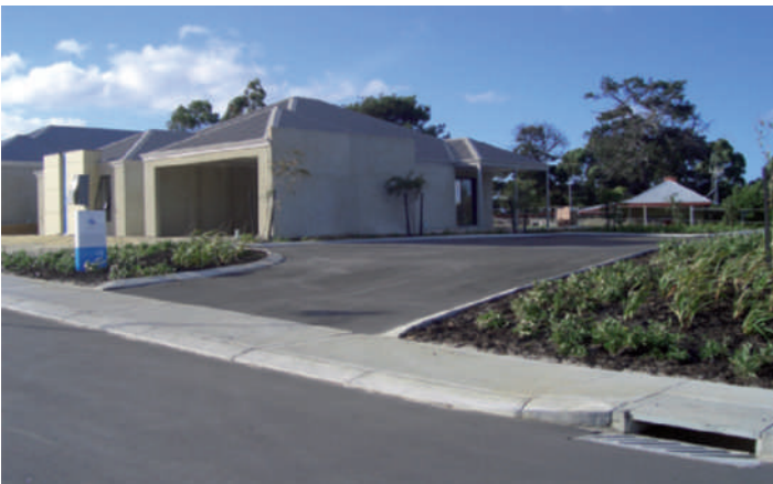
Y Garden bed mulched and planted soon after construction
