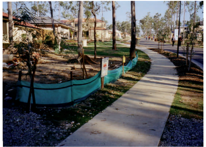
Y Good site planning – includes sediment containment fence
