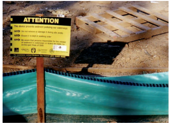
Y Correctly installed sediment fence
