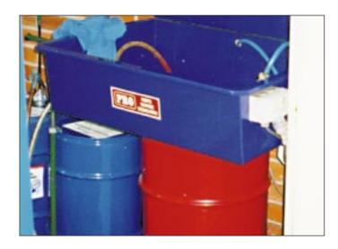
Store wastewater and washwater or waste cleaning solvents in tanks or drums to be collected by a licensed liquid waste transporter. This figure shows a solvent wash sink connected directly to the storage drum.
