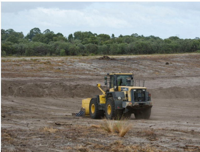
C. Topsoil harvesting at Jandakot Airport in April 2012. A thin 5 cm layer was harvested to maximise seed quantities, as most seed is near the surface.
