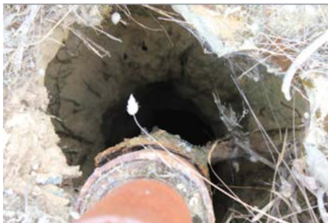
Figure 8. Picture shows subsidence around a tired 32 year old drill hole in the South East of South Australia, indicating that casings and cement are no match for geological processes in the short term, let alone over the next 100 to 1000 years.
