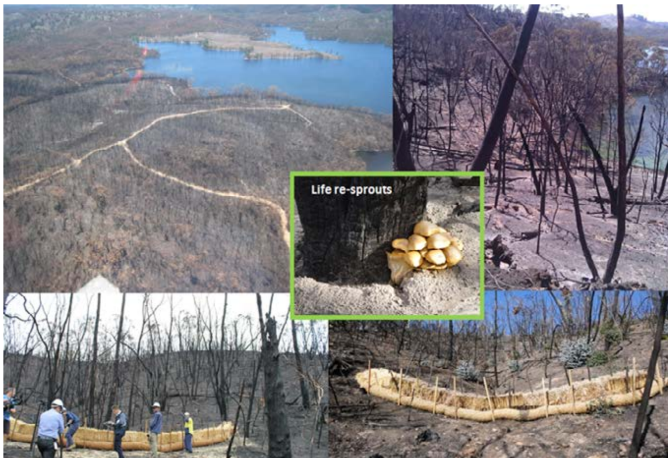
Figure 11. Installation of sediment control structures.
