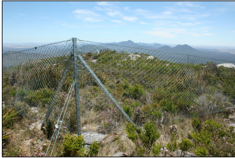
Figure 3. Corner straining box constructed of galvanized star iron pickets.
