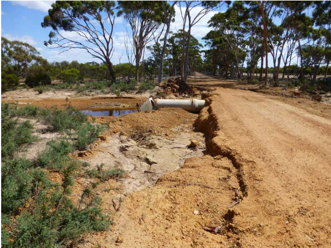
Figure 2. Severe erosion occurring on Brown Road, located immediately up-gradient from the West Drain (DWER site ID 609038), as a consequence of surface water flows occurring in February 2017.
