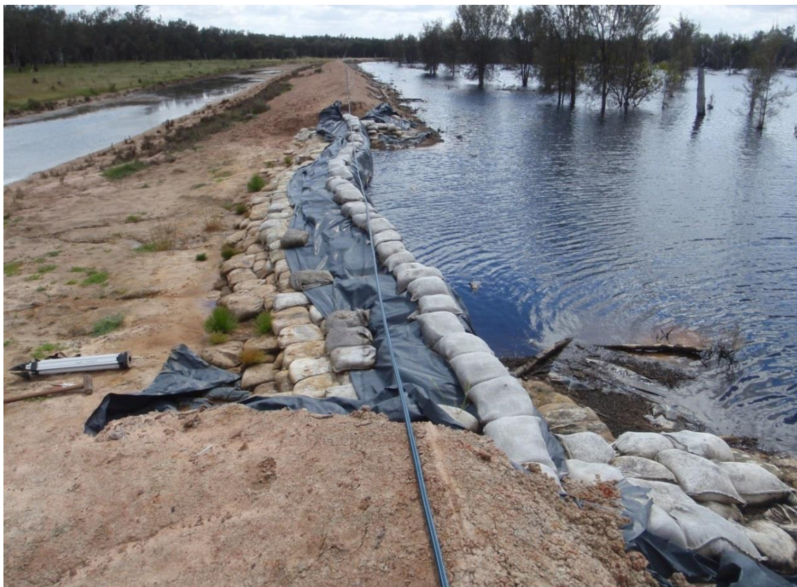
Figure 14. Northwards photograph of the repaired bund wall breach. Photograph taken on 18 October 2017 by Lindsay Bourke.
