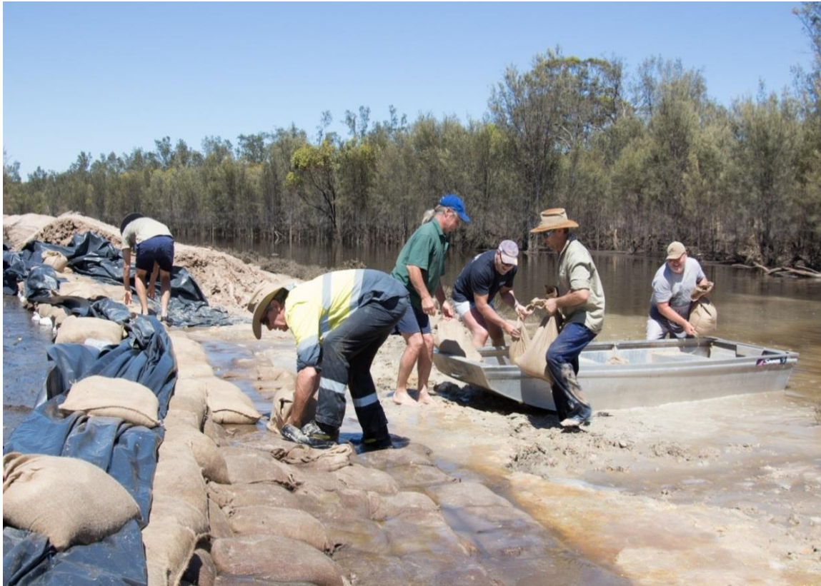
Figure 13. Repair of the Toolibin Lake bund wall breach being undertaken by DBCA staff and volunteers on Thursday 16 February 2017. Photograph by Maria Lee.
