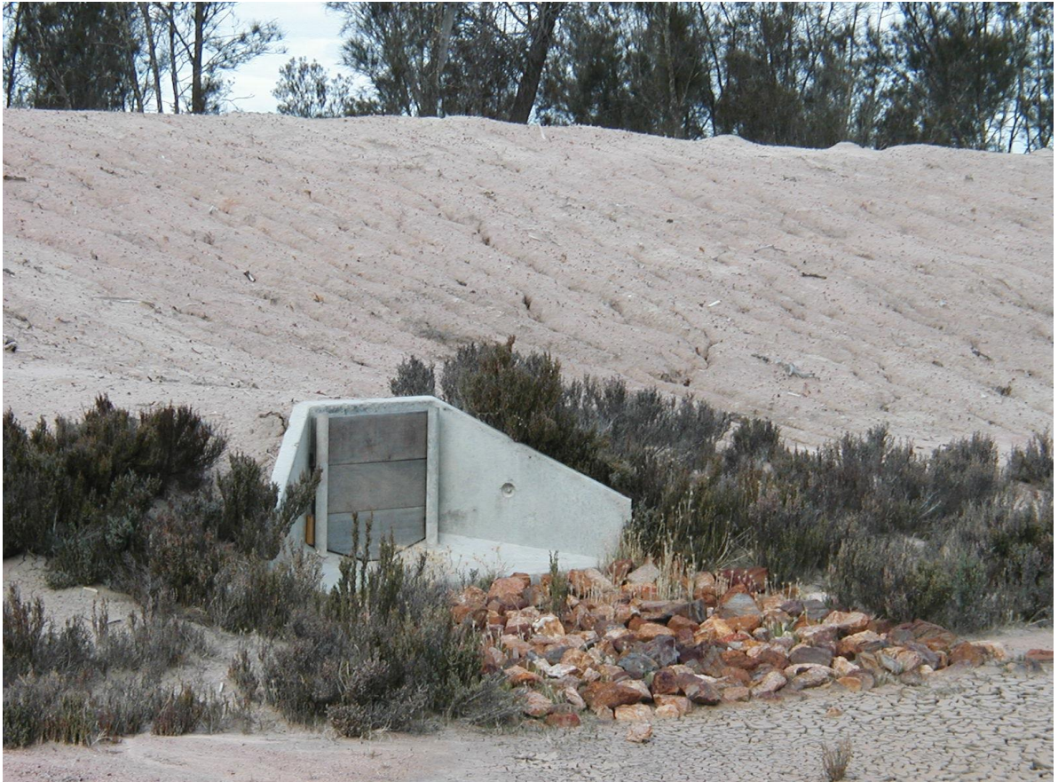
Figure 7. Photograph of the constructed lake outlet control
