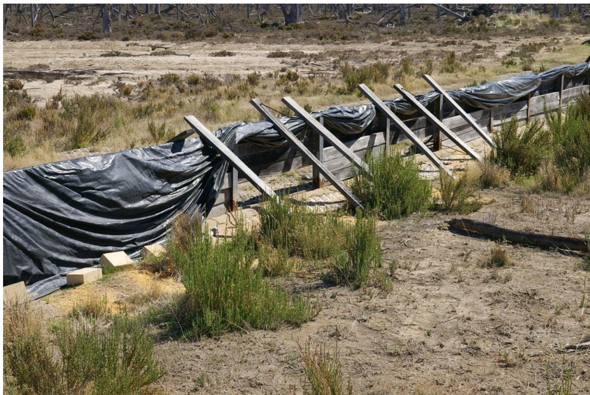
Figure 4. The original Toolibin Lake separator gate infrastructure. Note the lower boards were removed in two of the panels in the photograph. Photograph was taken in April 2010, prior to
