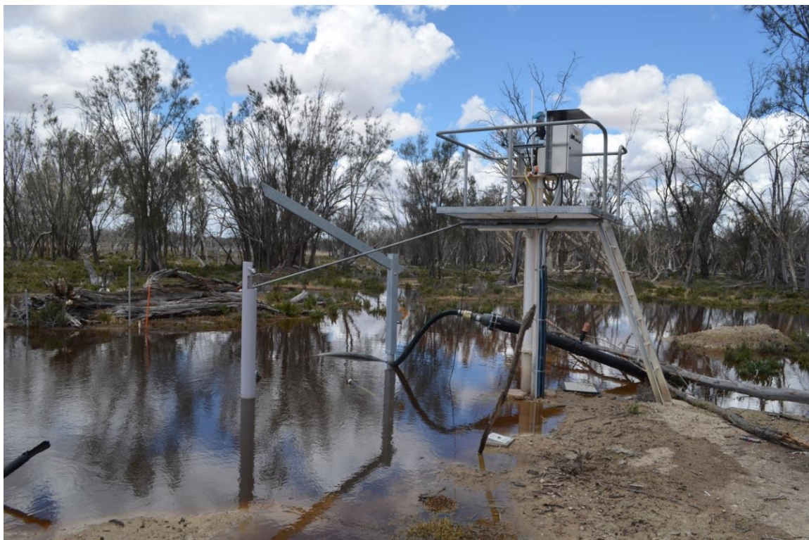
Figure 8. Sump fitted with gantry and pump (former Pump 8 and surface water monitoring site E)
