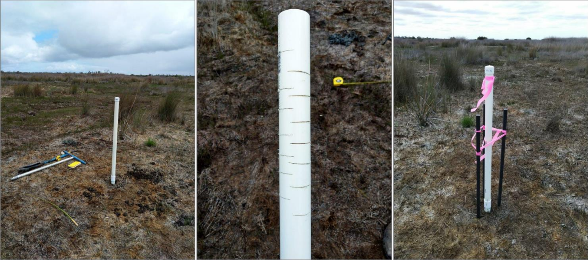
Transect 2 site TGN9b – mini piezometer construction, showing stick-up and screen slots
