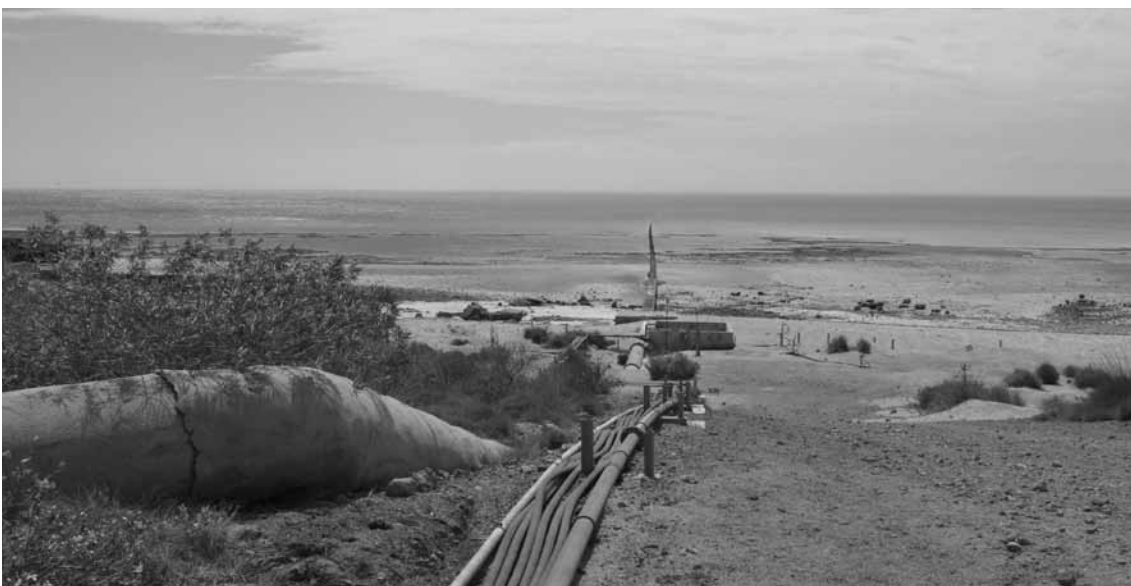
A significant amount of infrastructure exists on Barrow Island Nature Reserve including this tanker loading pipeline shore crossing on the east coast, near Town Point – Photo Kevin Crane (DEC)
