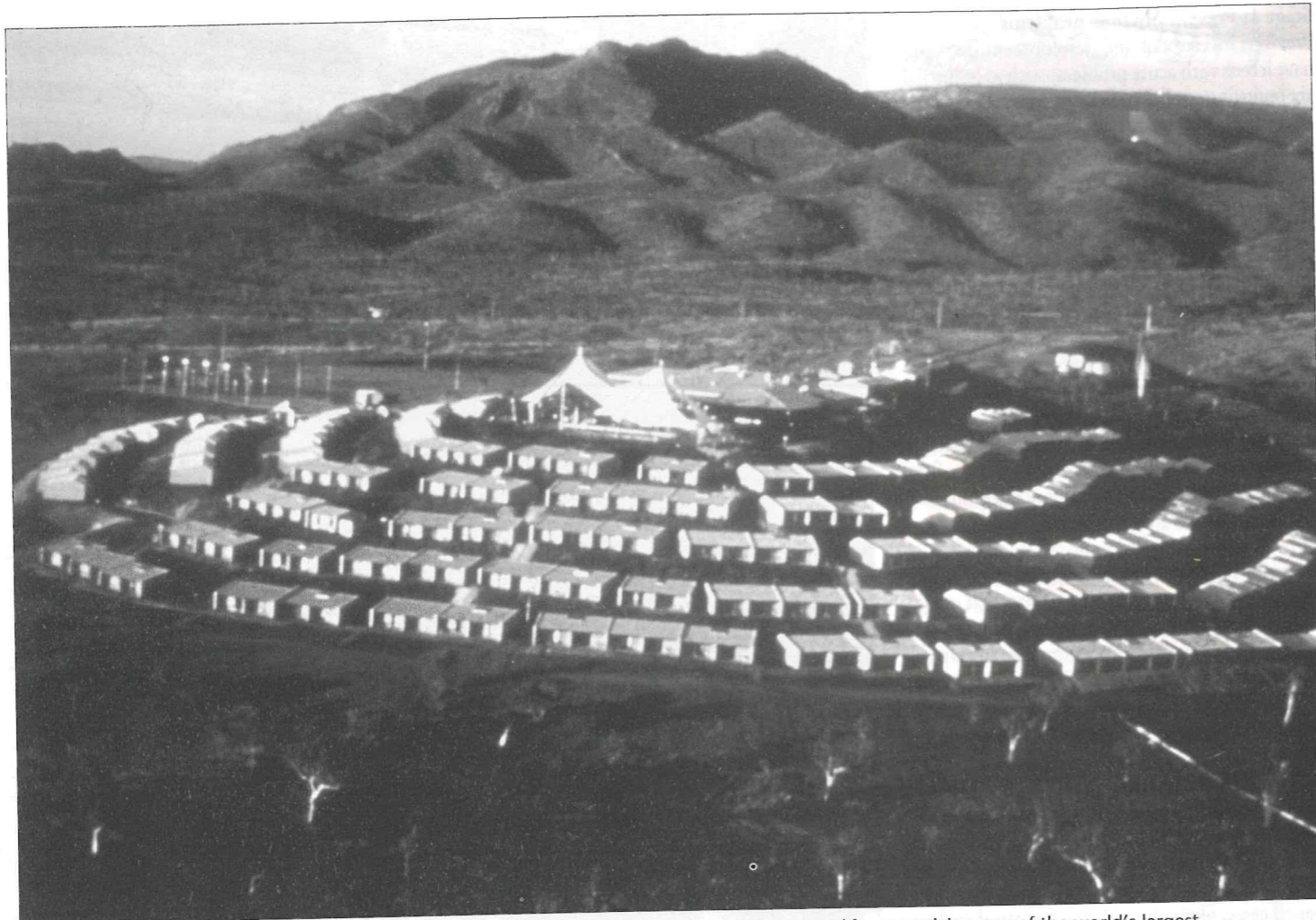
Lake Argyle area, Western Australia: Housing development for the commuter workforce servicing one of the world's largest diamond mines at Argyle. The fly in/fly out arrangement for the mine workforce reduces local environmental impact by avoiding the need to establish a full-scale urban community to service the mine. (Argyle Diamonds)
