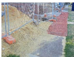
Figure 79: Skudo All-Terrain Mat in-situ at the City of Stirling. Photograph courtesy of Perth NRM.
