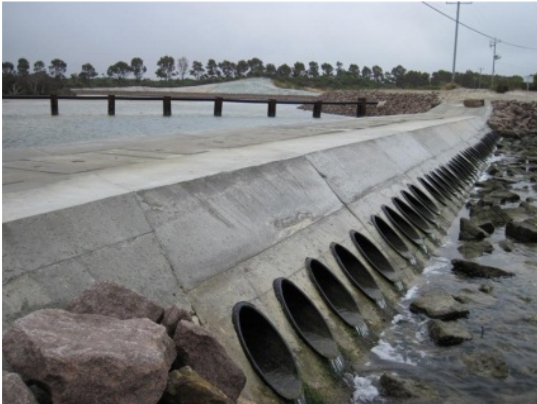
Figure 7. Current Bandy Creek weir.
