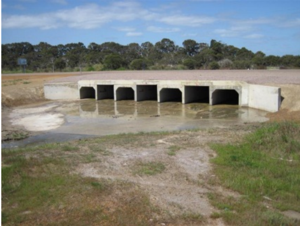
Figure 13. Fisheries road 'flow barrier' upgrade at Lake Wheatfield.
