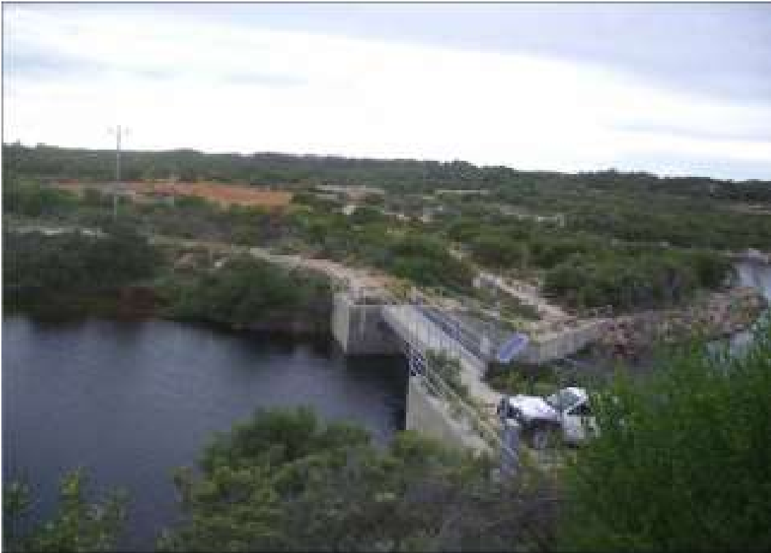
Figure 5. Bandy Creek weir before 2007 flood (Photo by Tilo Massenbauer).
