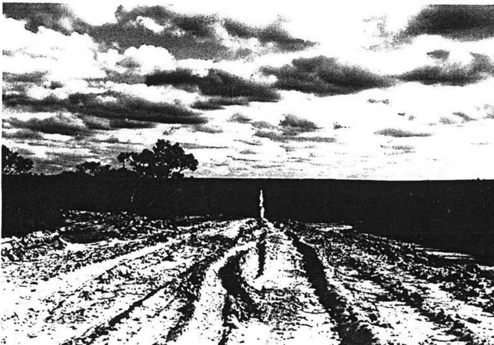
AS WELL AS THE POOR CONDITION OF THIS TRACK NOTE HOW THE TRACK IS VISIBLE FOR SEVERAL KILOMETRES BECAUSE OF STRAIGHTNESS
