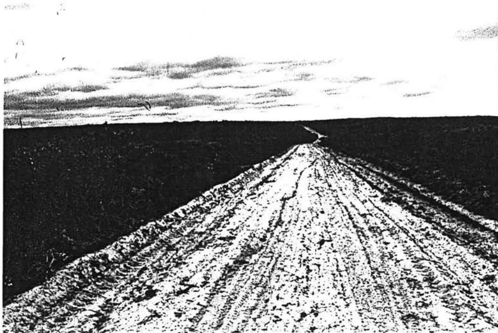
AN ALIGNMENT FOLLOWING CLEARING PRIOR TO FORMING
