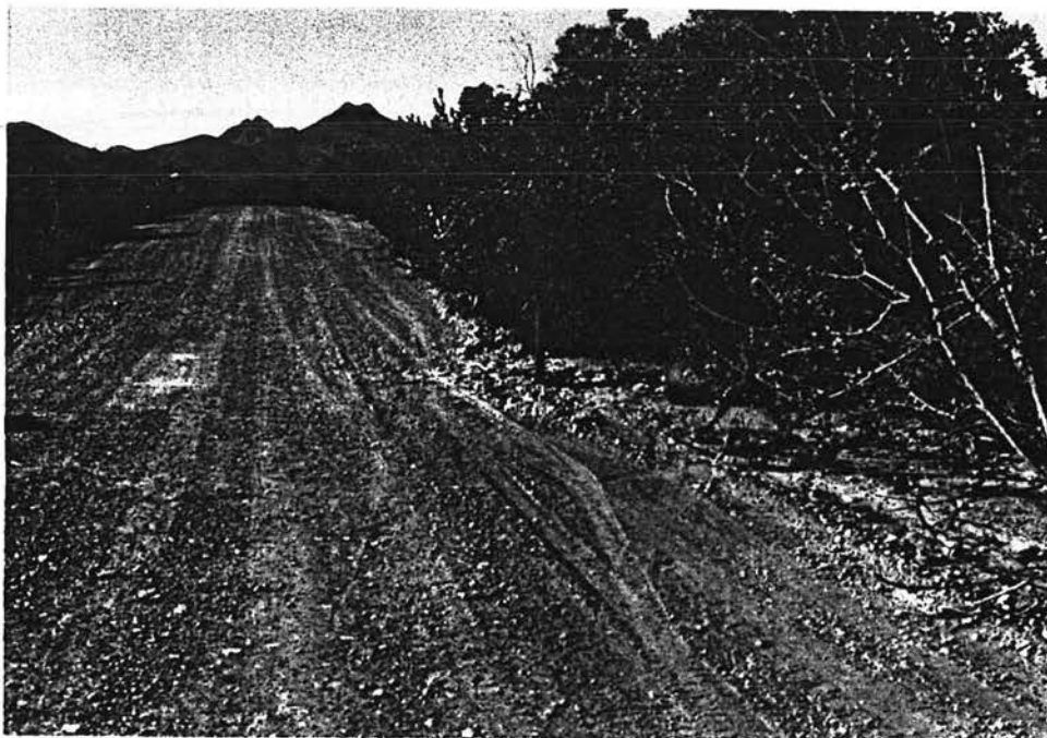
THIS SHOWS THE LACK OF A DRAIN CHANNELLING RUN OFF INTO THE CULVERT PROVIDED
