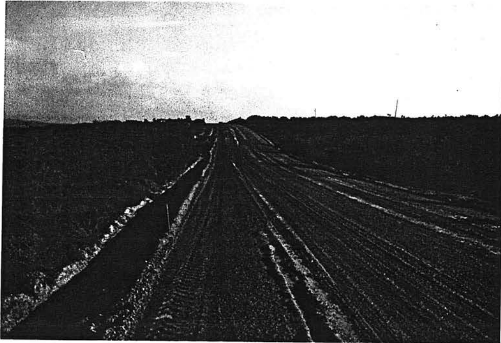
CAPE LE GRAND ROAD DURING THE EARLY STAGES PRIOR TO BITUMIZING
