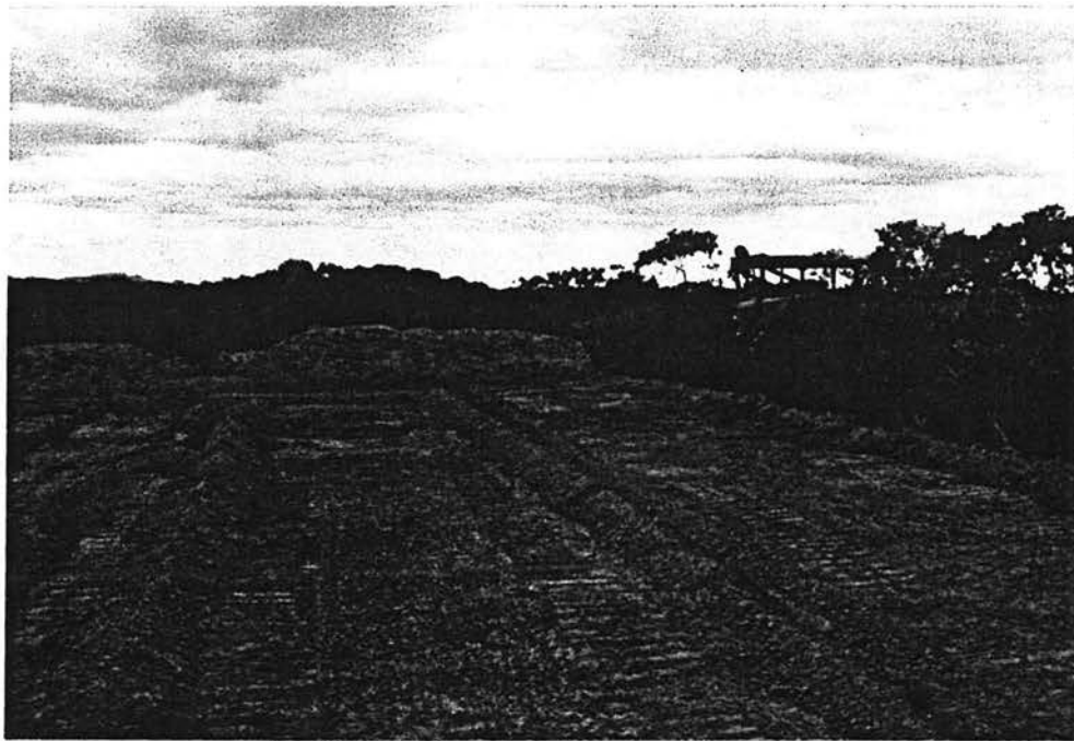
THE STRIPPING OFF OF THE TOPSOIL AND VEGETATION PRIOR TO GRAVEL REMOVAL
