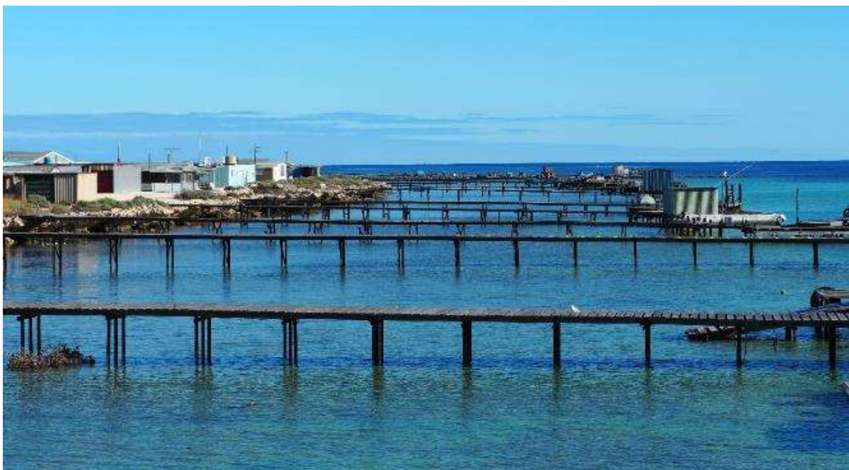
Fishing camps and jetties within Reserve 20253 are private property. There is no public access to these areas and facilities. Photo – Nathan Greenhill/DBCA
