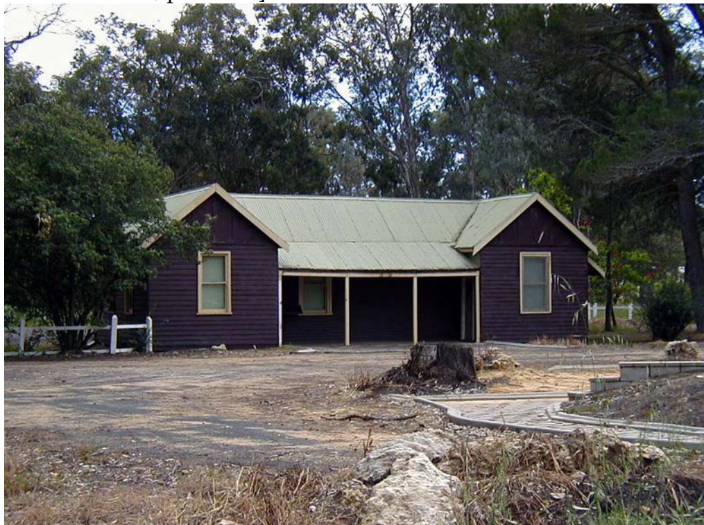
Photo 22 Building 42 - District Office [c1920s and c1957]
