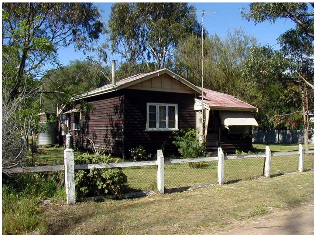
Photo 10 Building 855 - Forestry Cottage Type 8d [c1950]
