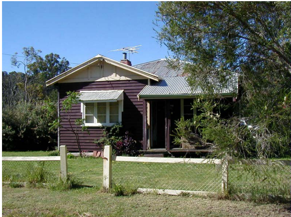
Photo 9 Building 853 - Forestry Cottage Type 8d [c1950]
