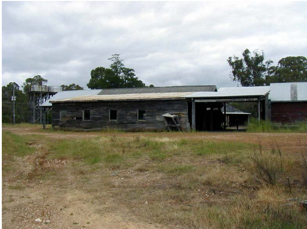
Photo 25 Buildings 939 - Planer Mill Building [c1950]
