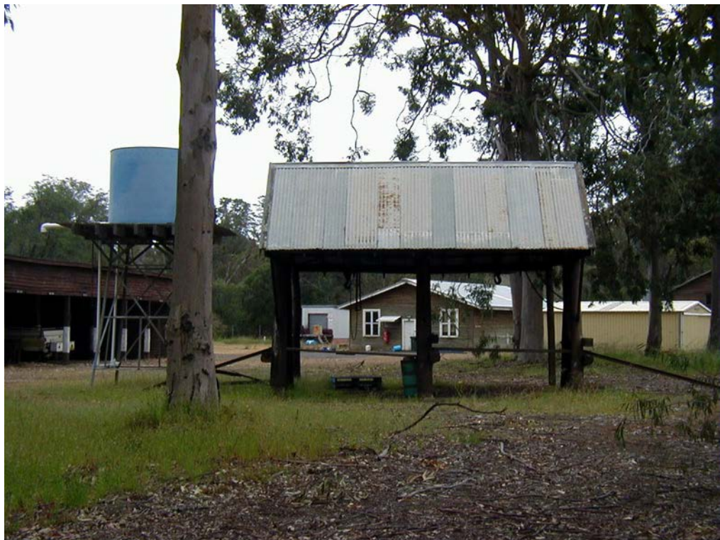
Photo 28 Building 1777 - Gantry [1960s]
