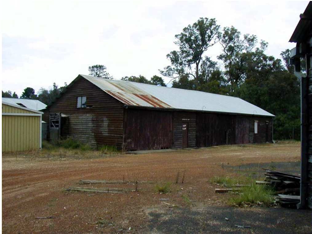
Photo 23 Building 654 - Workshop-Garage [c1950]
