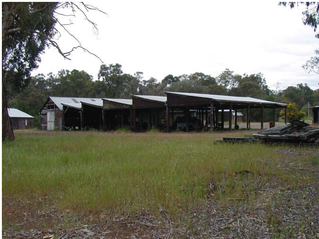
Photo 26 Buildings 940 - Timber Storage Shed [c1950]
