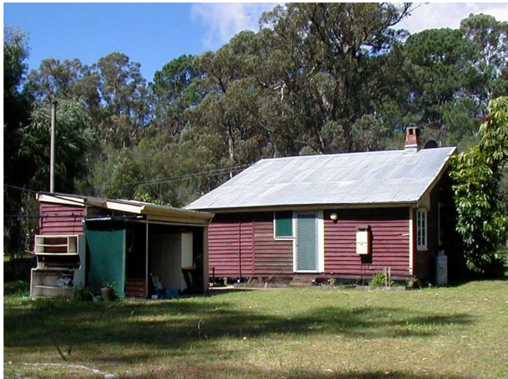
Photo 14 Building 625 (rear) - Forestry Cottage Type 8 [c1950]
