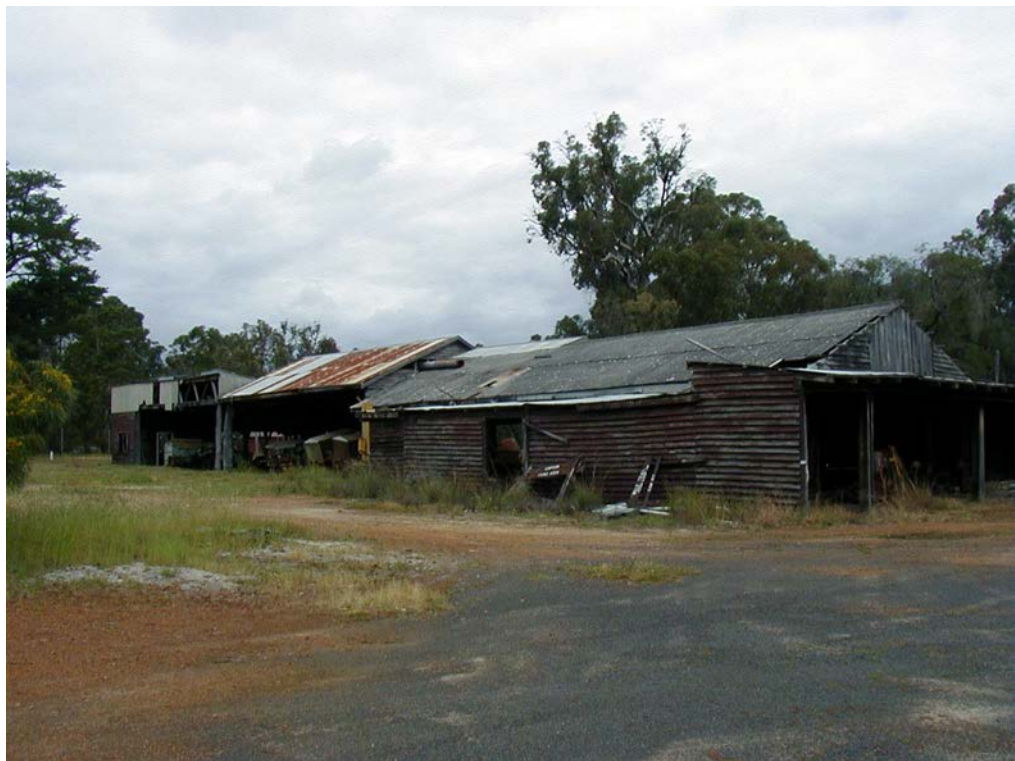
Photo 24 Building 655 - Sawmill Building [c1950]
