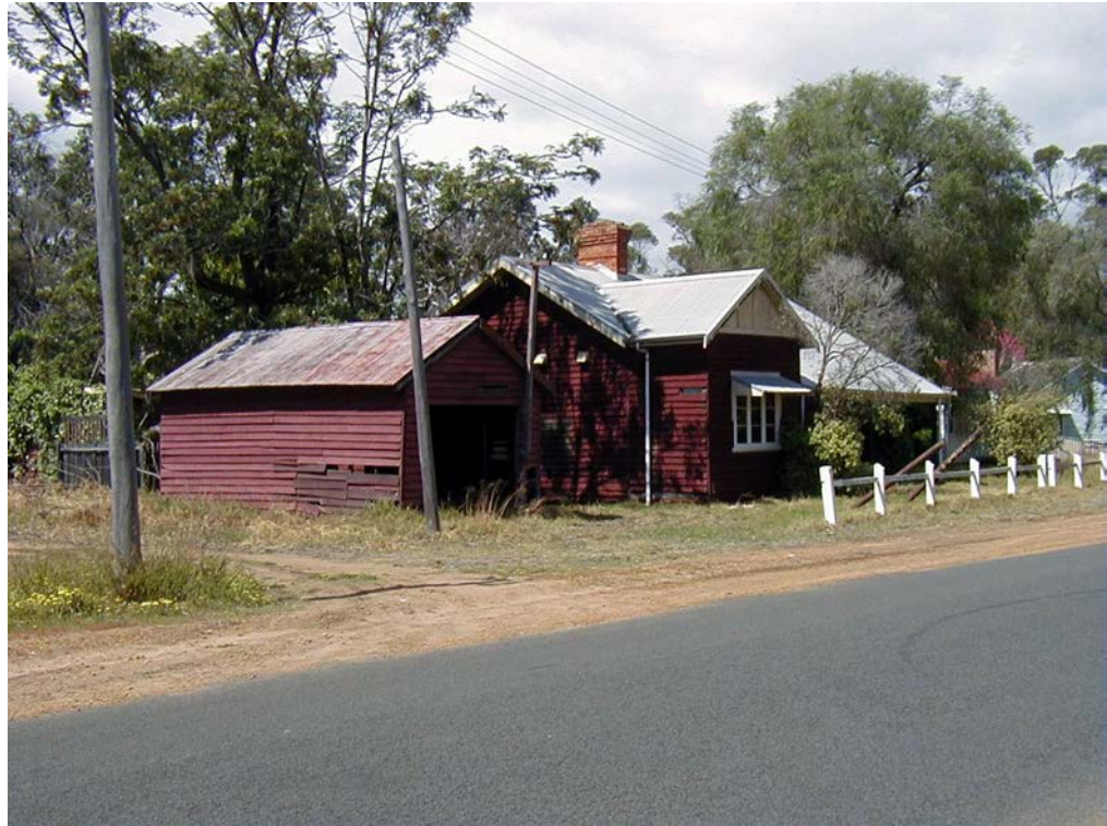
Photo 17 Building 680 - Former Education Department House [c1925]
