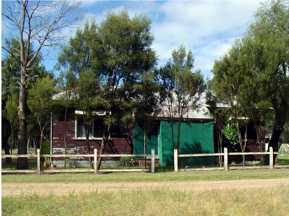
Photo 11 Buildings 1109 - Forestry Cottage Type 5 [1956]
