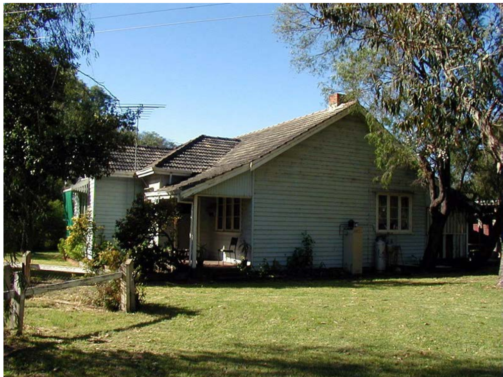
Photo 18 Building 711 - Forestry Cottage Type 6c [c1950]
