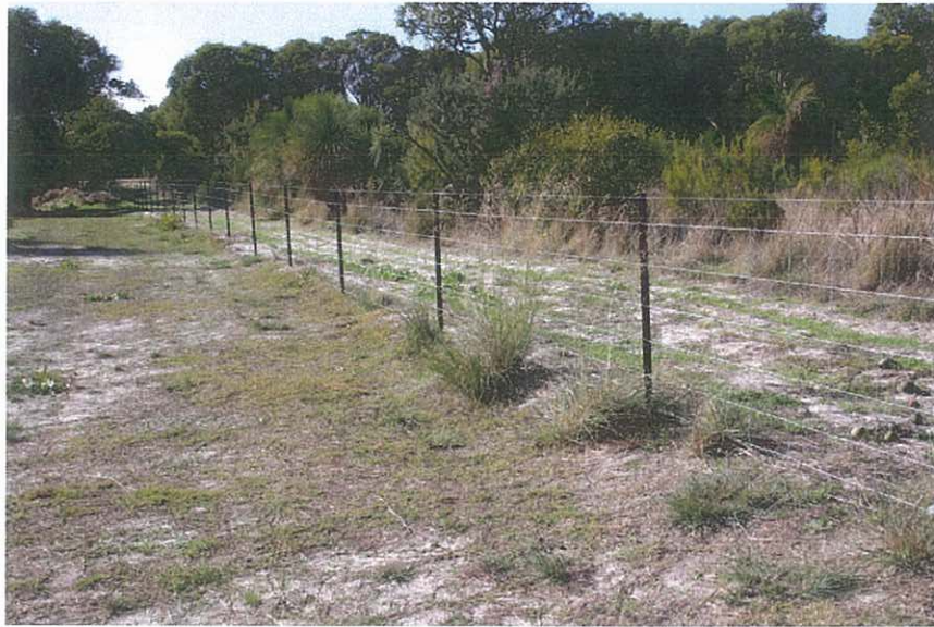
Installation of new fence along northern boundary Muchea Nature Reserve, Muchea
