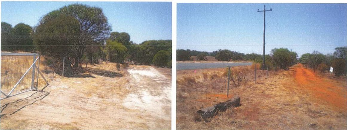
The new northern boundary fence installed at Timaru Nature Reserve
