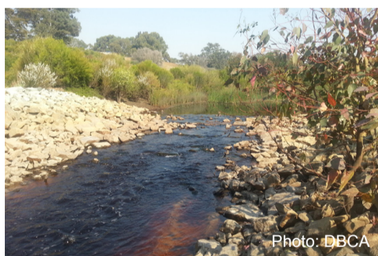
A riffle installed in Ellen Brook, October 2016.
