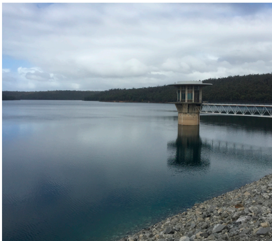
Helena River Pumpback Dam, August 2017. Photo: Emma van Looij
