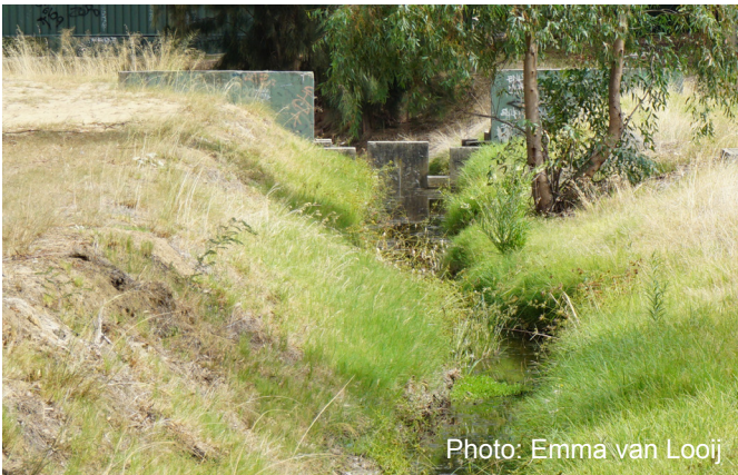
A flow control structure in Helm Street Drain, March 2016.
