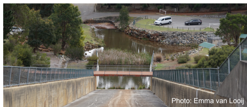
The spillway at Churchman Brook dam which is just upstream of the Upper Canning catchment, August 2017.
