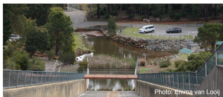
The spillway at Churchman Brook dam which is just upstream of the Upper Canning catchment, August 2017.
