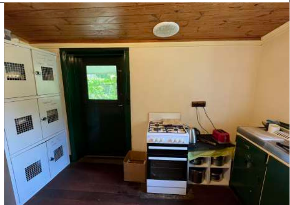
Kitchen eastern wall
