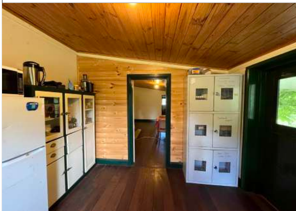
Kitchen partition wall
