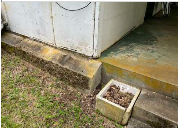
South elevation foundation
