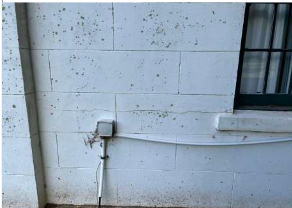
Conduit to northern organ room wall
