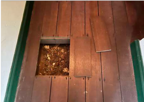
Original timber floor to hallway
