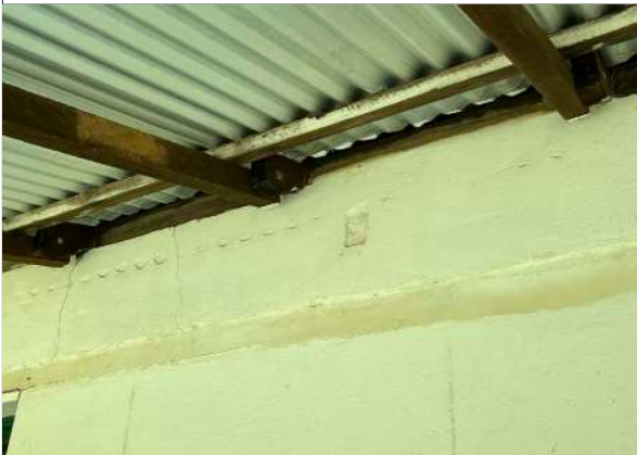
Wall connection showing previous location
