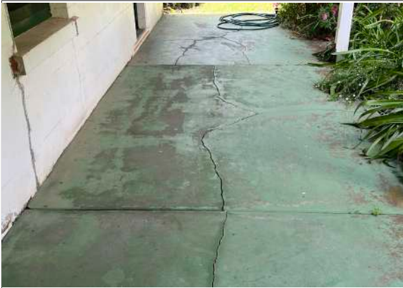
Front verandah slab
