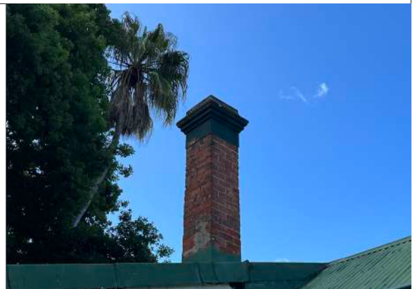
Chimney to organ room
