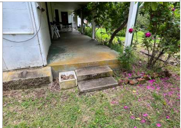
Southern steps to rear verandah
