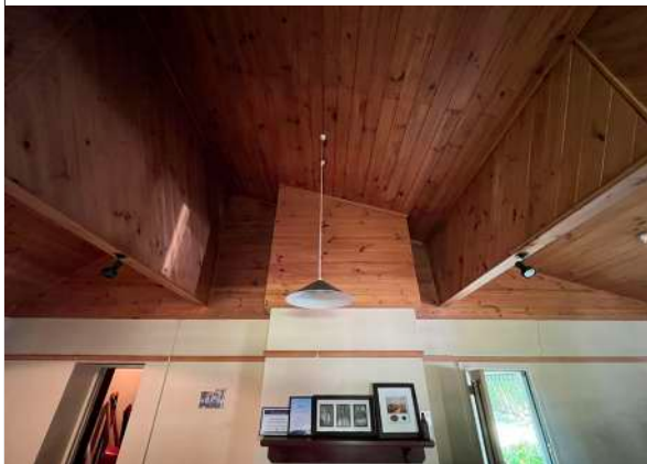
Organ Room roof structure
