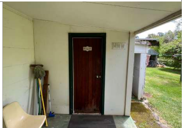
Bathroom built into verandah
