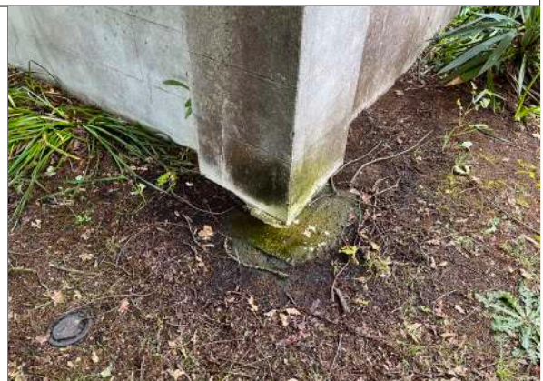
North-west corner pier foundation
