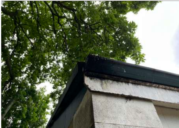
North -west organ room corner gutter
