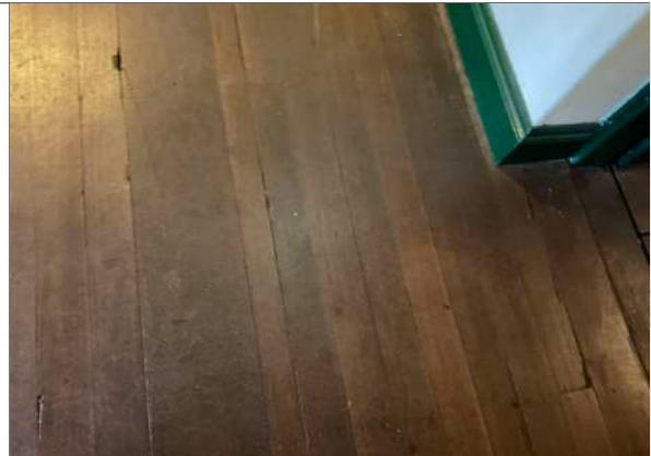
Replaced floorboards to Dining Room
