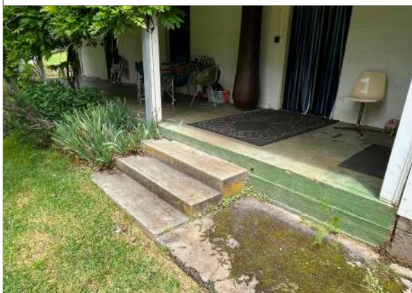
Northern concrete stairs to rear verandah
