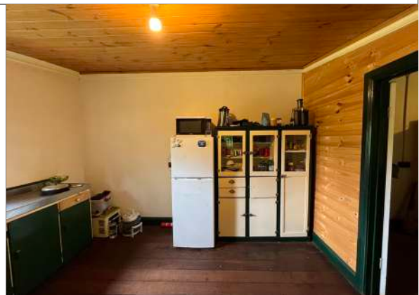
Kitchen western wall
