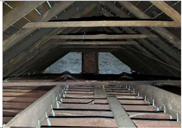
Bricked in window to northern gable
