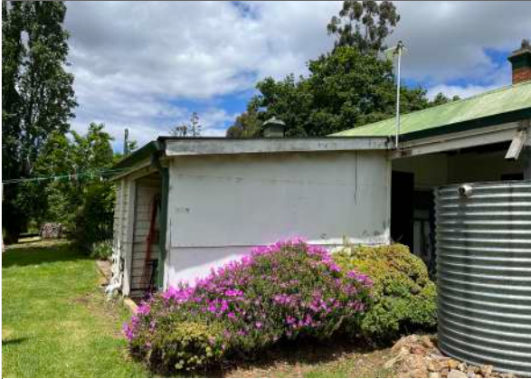
Shed/ Laundry to north corner
