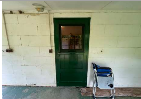
Door to Kitchen
