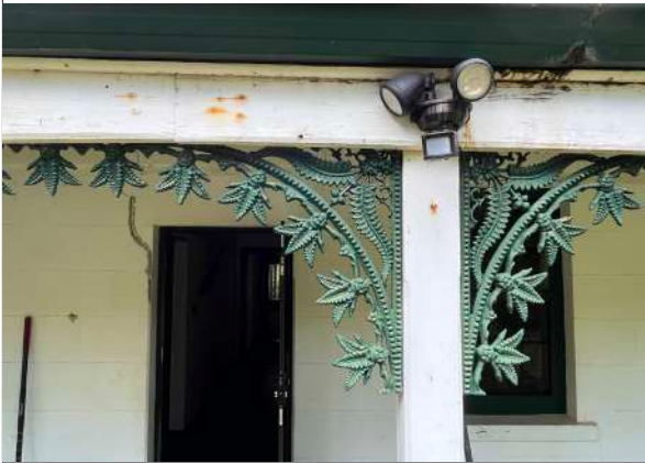
Front verandah post and frieze brackets
