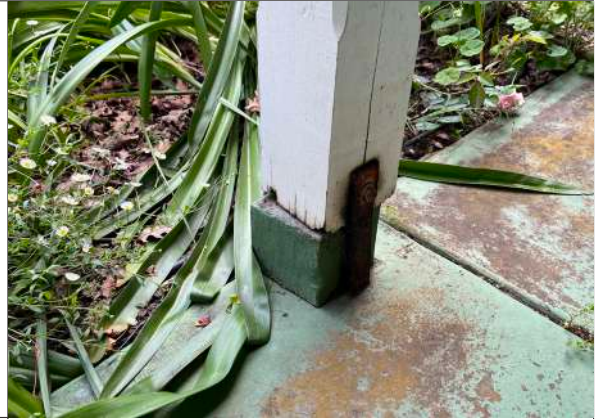
Front verandah post connection
