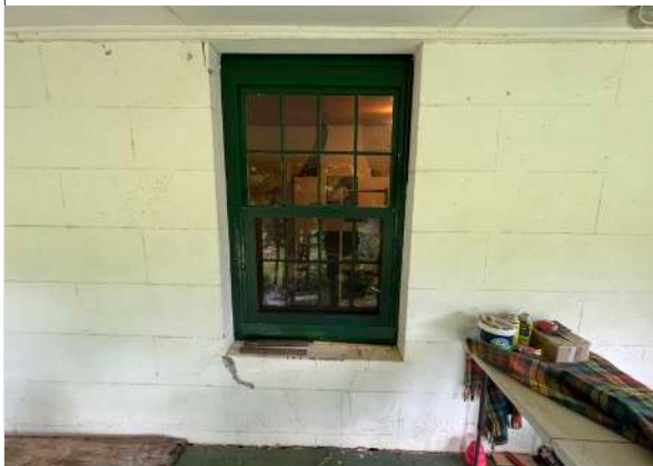
Window to dining room (W6)
