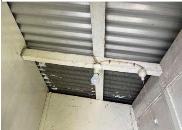
Toilet roof structure
