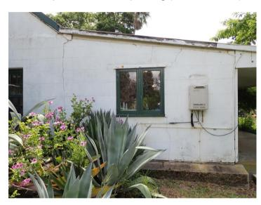
• There are other historic actions that have affected the early brickwork of this elevation - some differential settlement and some historic lintel steel corrosion. action. Past repairs have taken place and some reopening of crack has occurred. The step in the wall face between lower brickwork and triangular loft gable panels is not a wall movement, it reflects a change in construction from 9" to 4.5" brick.
