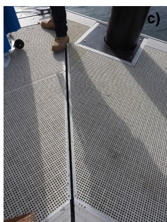
Figure 33. Aluminum edging used on Jetty 2 at the Swan Yacht Club (a), South of Perth Yacht Club (b), and Swan Yacht Club pontoon (c) protected fibre reinforced decking from wear in comparison to an example where edging is recommended (d - John Tonkin Reserve beach access ramp).
