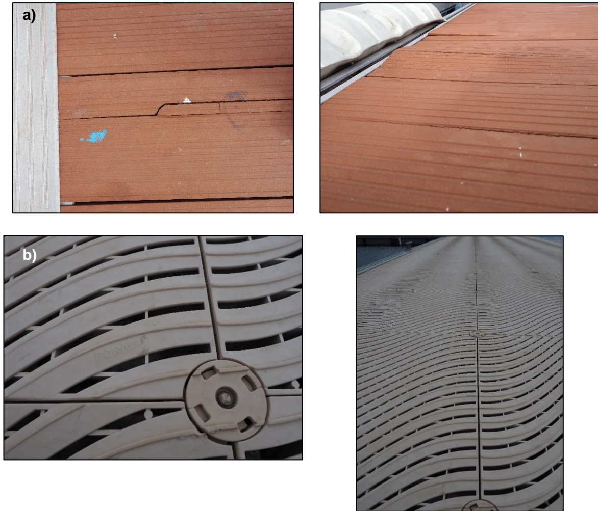
Figure 26. Other types of plastic decking observed including composite plastic at the South of Perth Yacht Club (a) and hard plastic decking (most likely polypropylene) at the Perth Flying Squadron Yacht Club (b).
