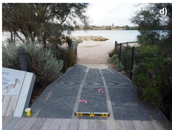
Figure 33. Aluminum edging used on Jetty 2 at the Swan Yacht Club (a), South of Perth Yacht Club (b), and Swan Yacht Club pontoon (c) protected fibre reinforced decking from wear in comparison to an example where edging is recommended (d - John Tonkin Reserve beach access ramp).
