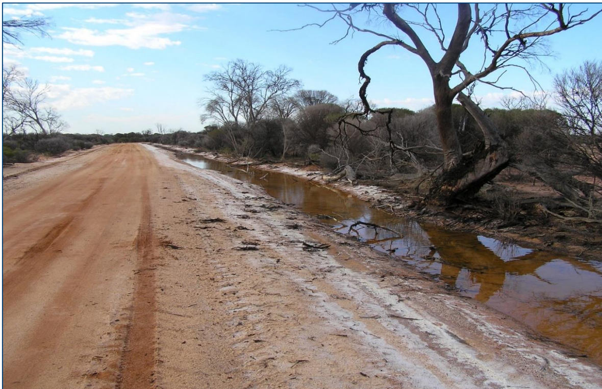
Figure 6: A local road in the eastern Wheatbelt showing damage; waterlogging and surface salt
