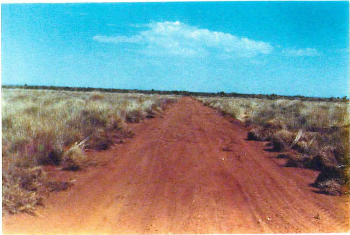
Fig. 1 Line cut with minimum removal of topsoil.
