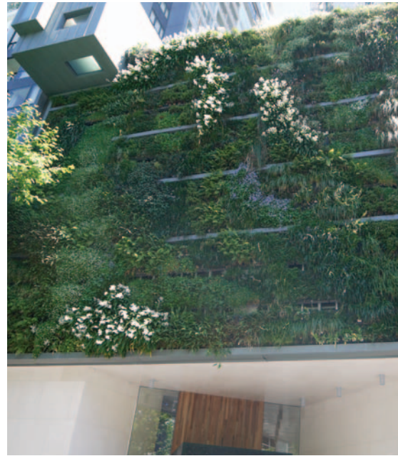
A vertical garden provides an attractive facade for a multi-storey car park in a large apartment block in Melbourne. Photo: Fytogreen Australia Pty Ltd.
