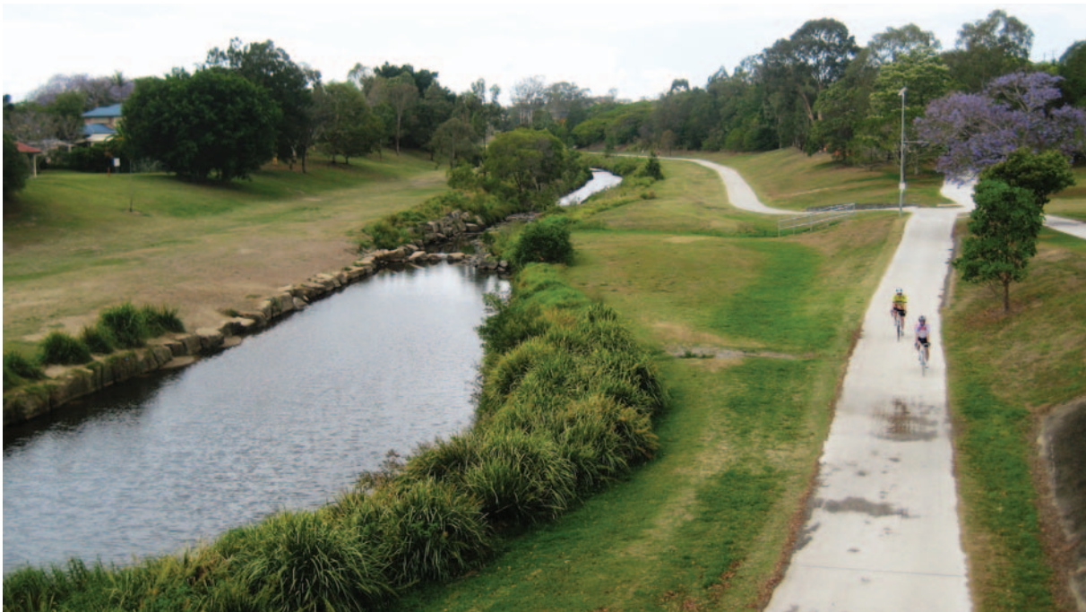
Green corridors can promote the movement of species into and around urban areas. This one follows Kedron Brook through Brisbane's northern suburbs, just 6 km from the CBD. Photo: Fiona Brown, CSIRO.
