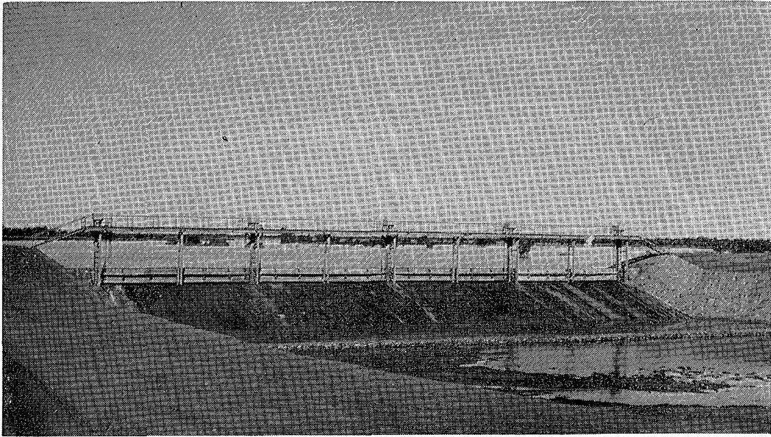
Spillway of 17 mile dam. Camballin.
