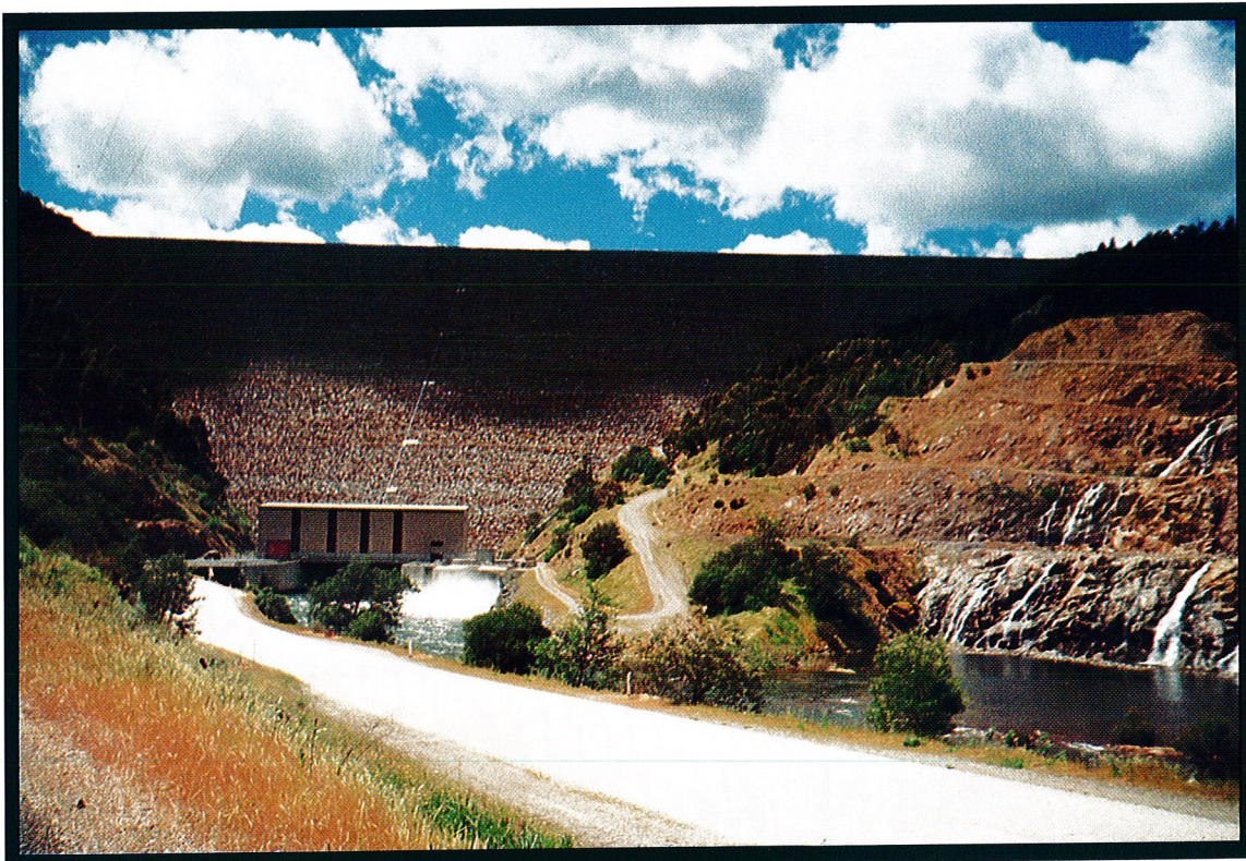
Dartmouth Dam, Spillway and Power Station
