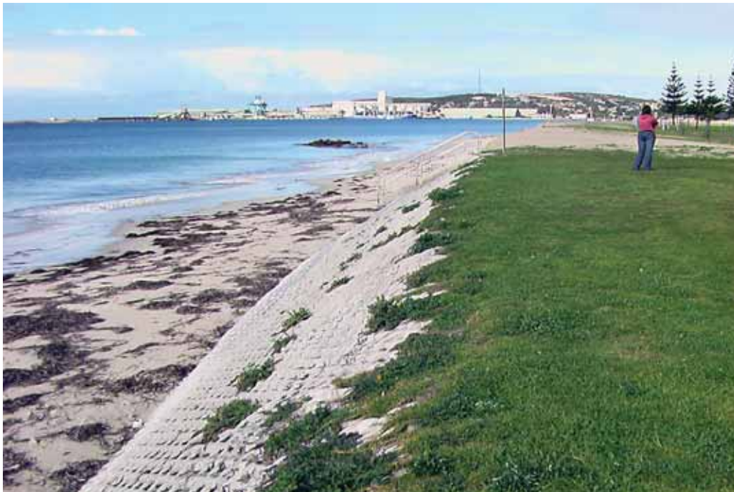
Jetty West Foreshore, Esperance
