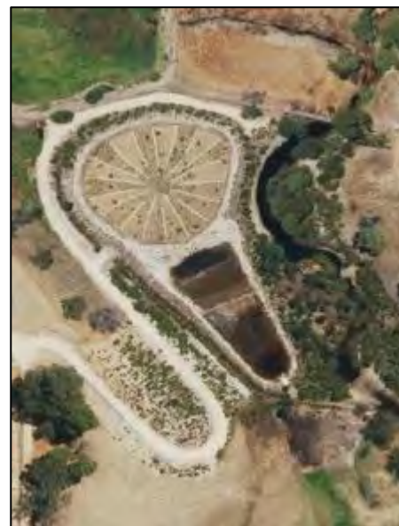
Aerial view - after construction
