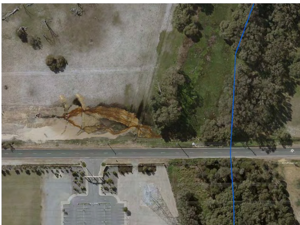
Figure 25: Sediment plume evident on the north side of the Marshall Road crossing.
