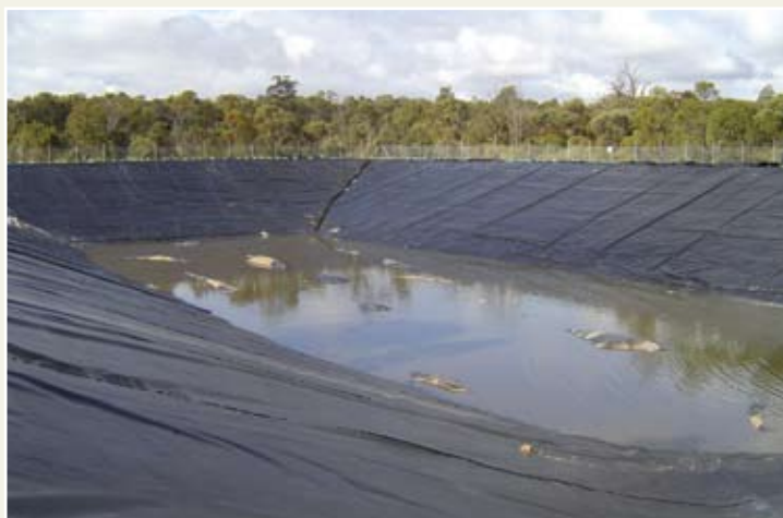
Photo 7 Plastic lined reservoir for wastewater and stormwater storage (Photo by Phil Steven)
