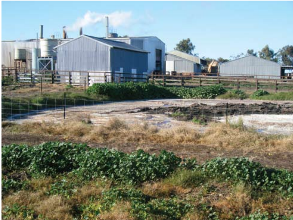
Photo 11 Anaerobic pond adjacent to the Avon Valley Beef meat processing plant (Photo by Viv Read)
