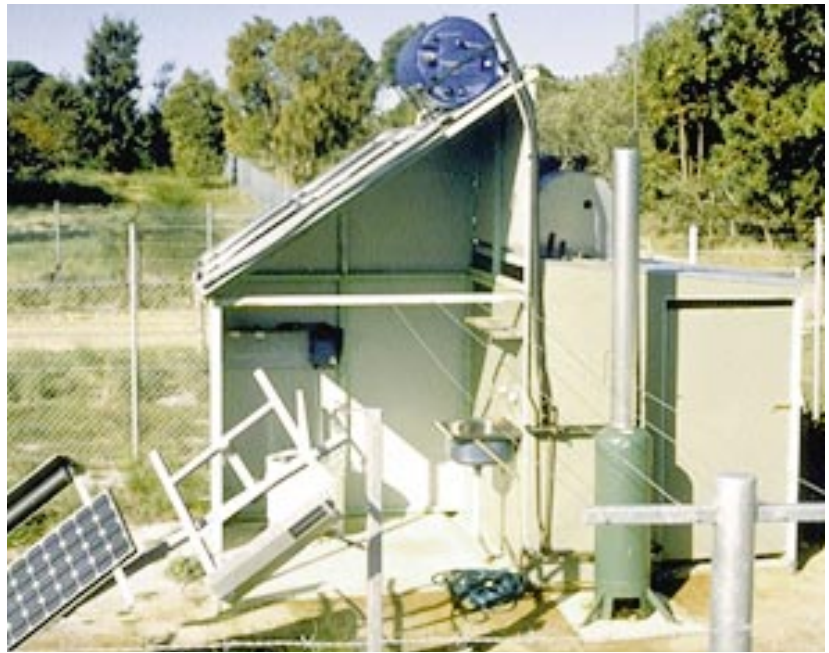
▲ Demonstration model of a remote area community ablation block with low-water-use toilet, wood and solar water heating, shower, hand-pumped washing machine and photovoltaics for electricity, if required.
