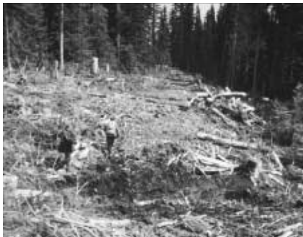
FIGURE 51 A view of the spur road following 2001–2002 logging. Note the narrow width of the road and right-of-way (D. Wilford photo).
