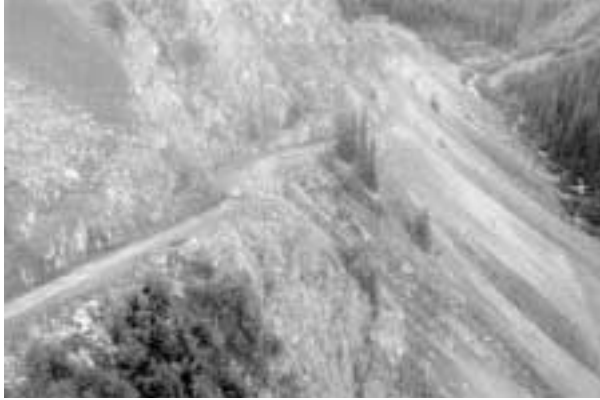
FIGURE 46 Looking south at the critical section of Option 4 following construction (C. VanBuskirk photo).
