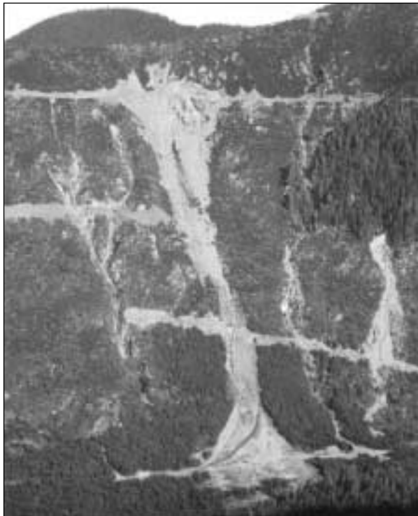
FIGURE 4 Example of a debris flow control structure (a deflection berm) near the base of the slope to protect fish habitat (M. Wise photo).
