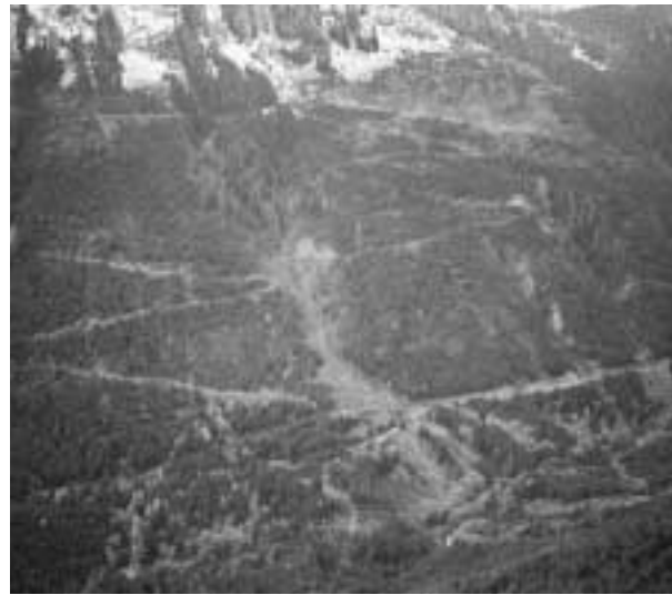
FIGURE 1 Steep slopes with branch roads, cutblocks, and gully areas above mainline forest road and utility corridors, coastal British Columbia (M. Leslie photo).
