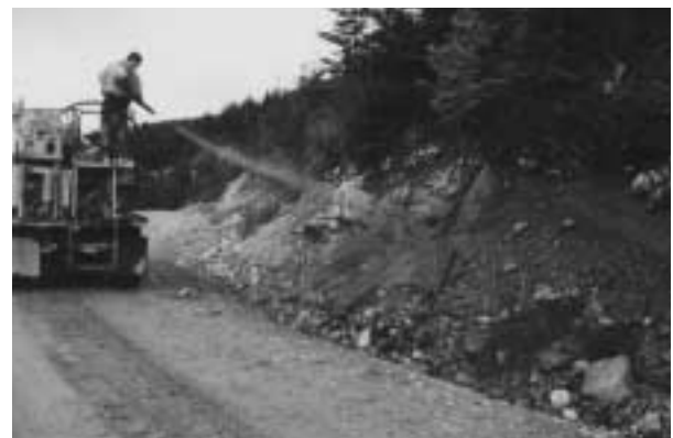
FIGURE 22 Hydroseeding exposed road cutslopes in the Lens Creek sub-basin (A. Hasanen photo).
