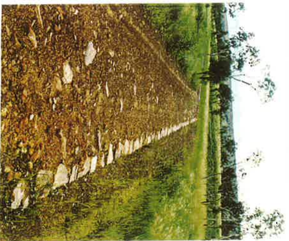
PLATE 1. COBBLESTONE EDGES OF 2 ND HALL'S CREEK ROAD
