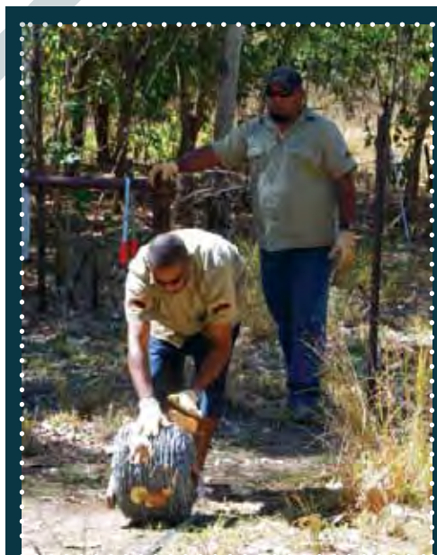
Miriuwung Gajerrong rangers, Jerimiah Hester and Chris Retsas, repairing the boundary fence of Point Springs Nature Reserve, adjacent to Jemarnde-wooningim, September 2008
