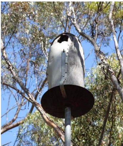
Figure 15: A crack in an artificial hollow repaired using a sheet of metal.
