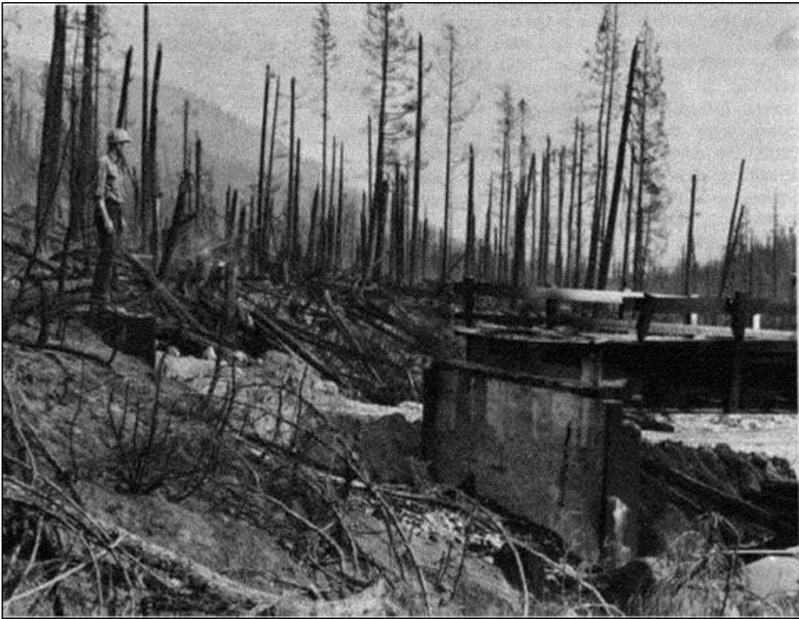
Dick Rothermel standing near the remains of the Pack River Bridge, destroyed during the major run of the Sundance Fire in northern Idaho (from Anderson 1968). On one day, September 1, 1967, 90 percent of approximately 56,000 acres (22,665 hectares) burned. Photo: William H. Frandsen, U.S. Forest Service, Intermountain Forest and Range Experiment Station, Northern Forest Fire Laboratory, Missoula, Mont. 1967.
