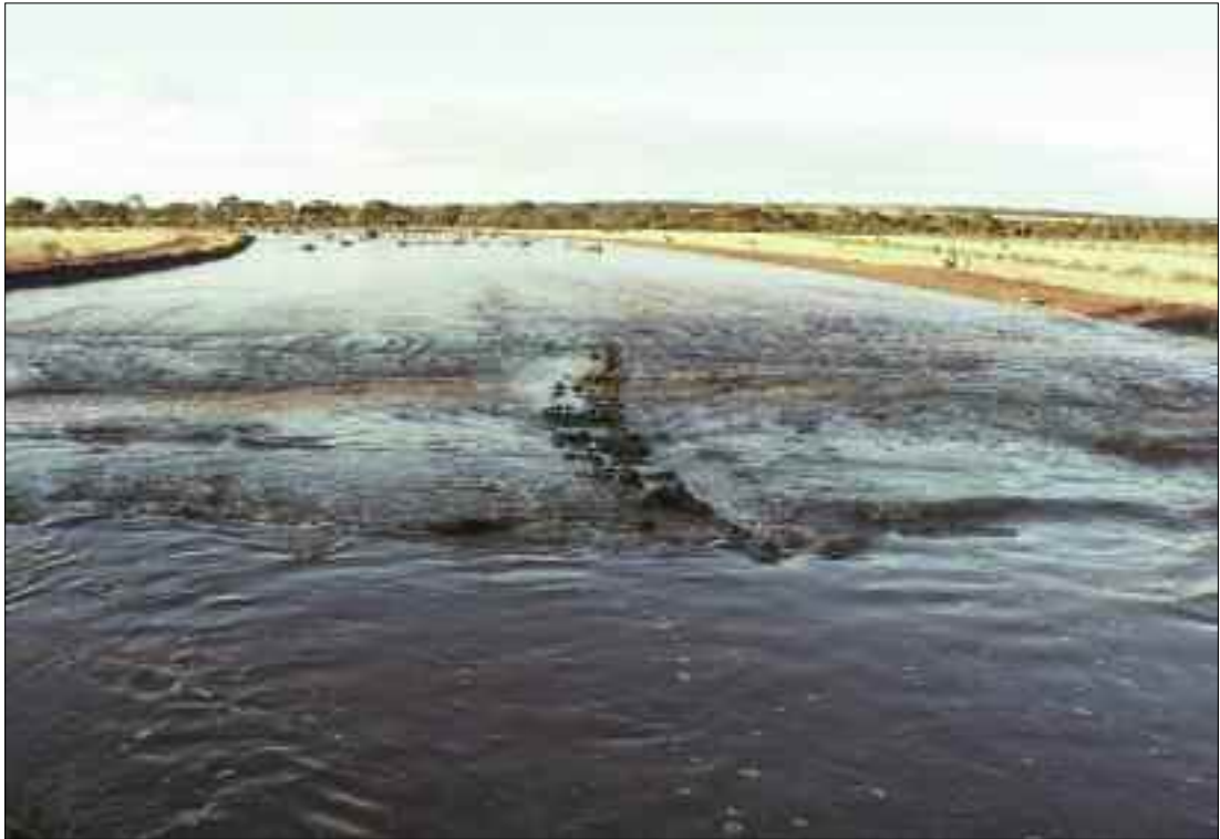
Photograph 2. Downstream from the new culvert, the constructed grassed waterway performed well in the one-in-45 year rainfall event. Photograph courtesy of Kathy Stone.
