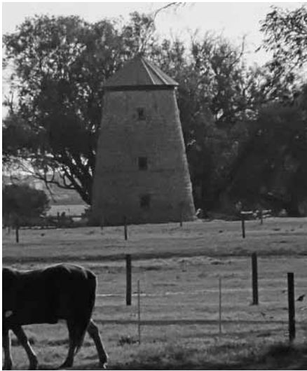
Former land use around the lime kilns. Photo – DEC
