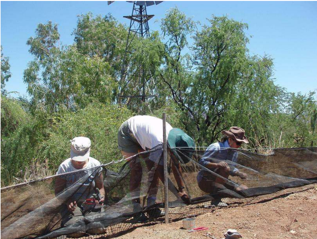
Volunteers attaching wildlife friendly gates to the exclusion fences to allow access by native animals, but not cane toads.
