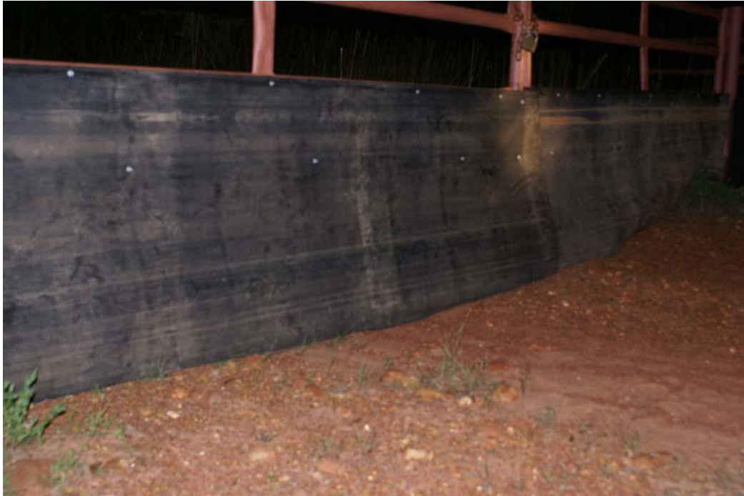
Rubber matting attached to gates can be effective as a barrier to toads
