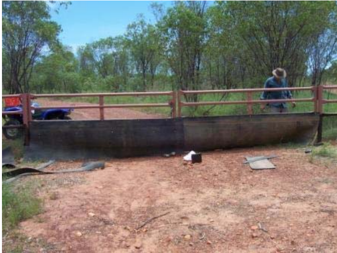
Attaching rubber matting to a gate to maintain barrier continuity
