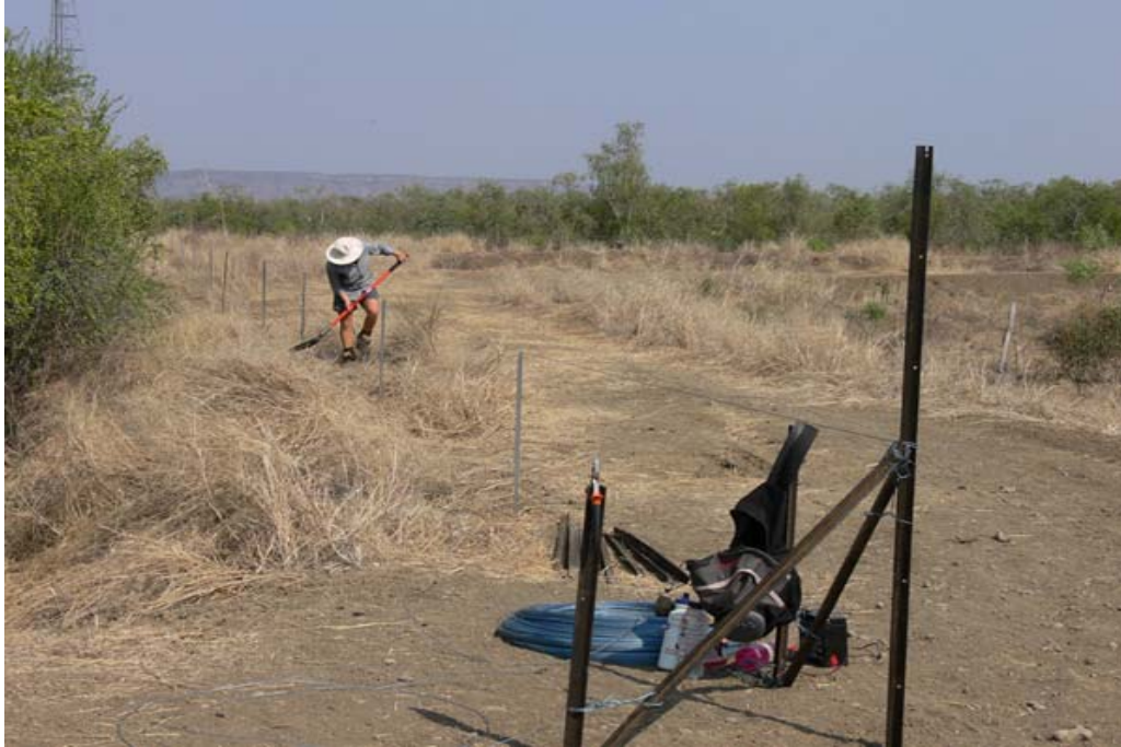
Fence corner assembly and wire showing dropper placement.
