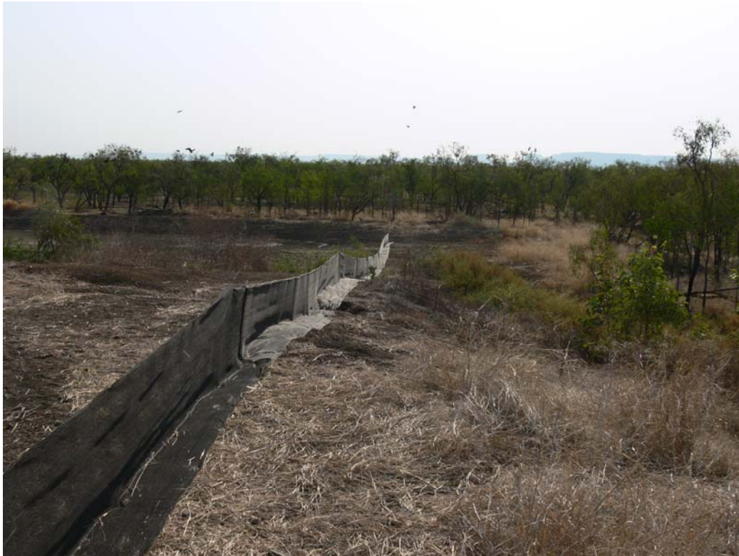
Cedars Lagoon fence showing the run down the northern bank to the overflow area (west). Note how the shade cloth is fitted to the contours of the ground.
