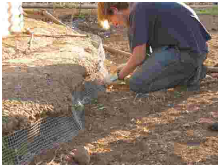
Volunteer erects temporary wire mesh around Ballinger tank.
