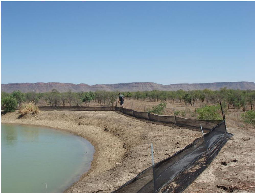
An example of a fence set up along the easiest route about 3m from the waters edge.
