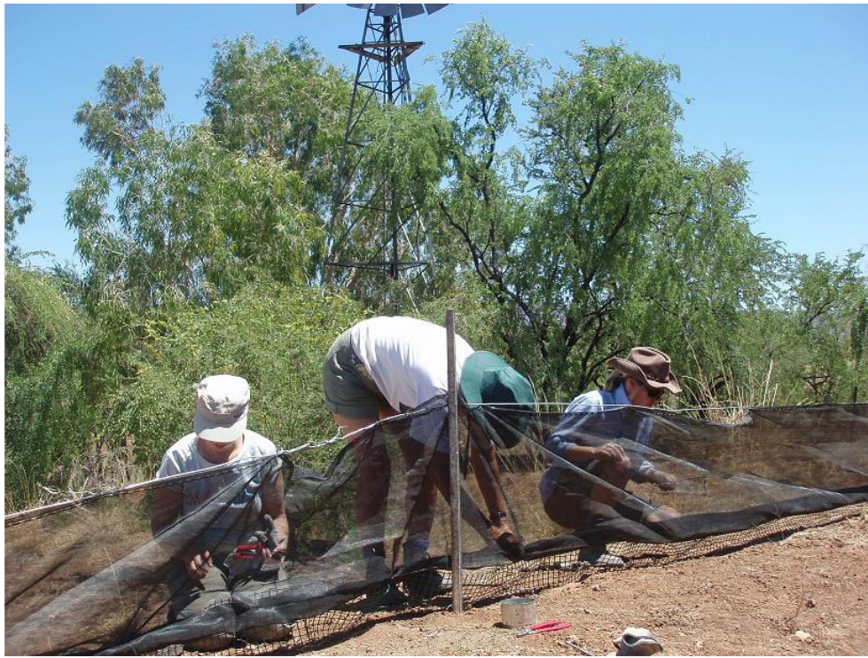
Volunteers inserting 25mm square mesh along the bottom of the fence as wildlife friendly gates.
