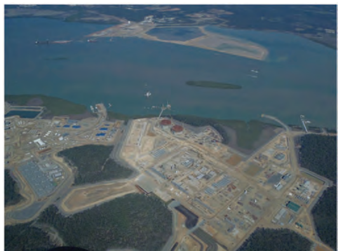
Photo: Curtis Island LNG port development, Gladstone, Queensland. (Teri Shore – SeaTurtles.org)
