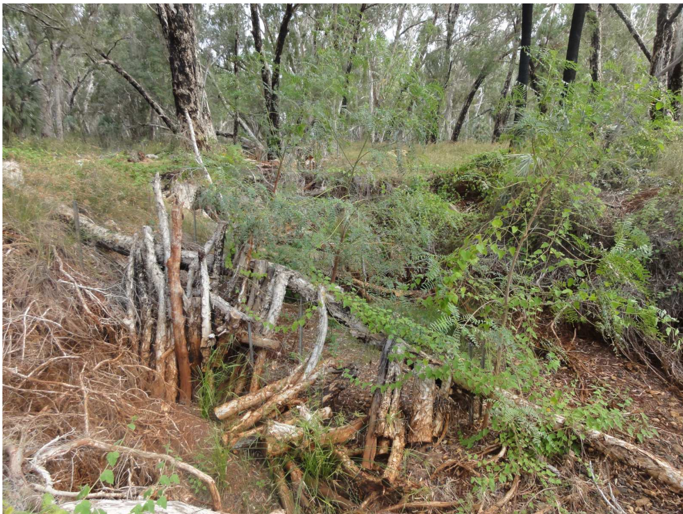
^^ Main erosion gully looking upstream toward headcut, July 15. Some collapse of log dam.
